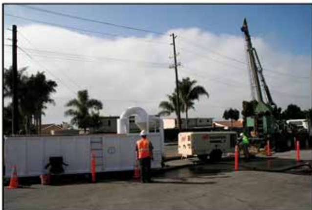
Figure 10. Redevelopment of the older injection wells requires heavy equipment and more time (left photo), whereas air-lift pumping of the newer injection wells can be done quickly using a mobile air compressor and dedicated sounding tubes (right photo).
