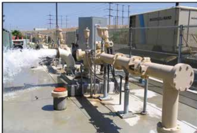
Figure 10. Redevelopment of the older injection wells requires heavy equipment and more time (left photo), whereas air-lift pumping of the newer injection wells can be done quickly using a mobile air compressor and dedicated sounding tubes (right photo).
