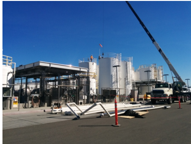
Feb 24 – Lifting Sulfuric Acid Piping
