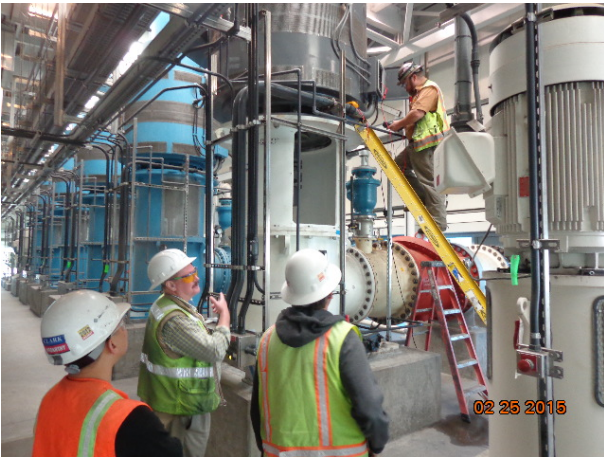
Jan 25 – Witness Testing ROTP Motor
