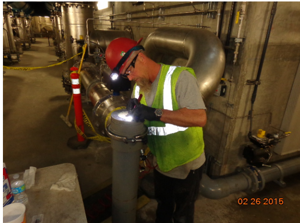
Feb 26 – Ongoing MF Membrane Pinning
