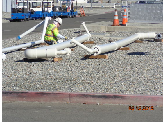
Feb 12 – Painting Sulfuric Acid Vent Piping
