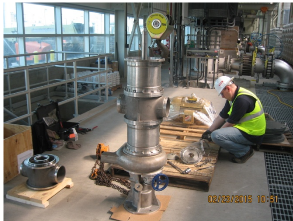
Feb 23 – Rebuilding F02 ERD
