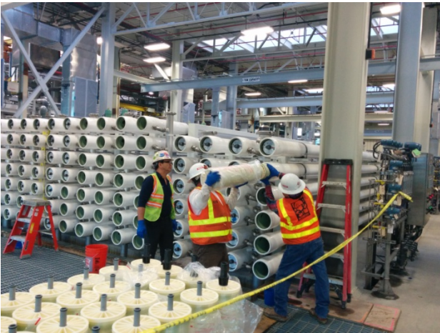
Feb 23 – Loading RO Membranes Unit F03
