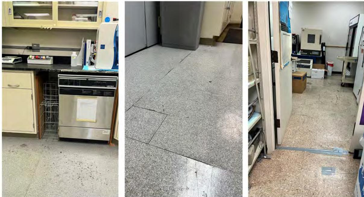
Figure 1: Various R&D laboratories' flooring features scuffing and general wear-and-tear.
