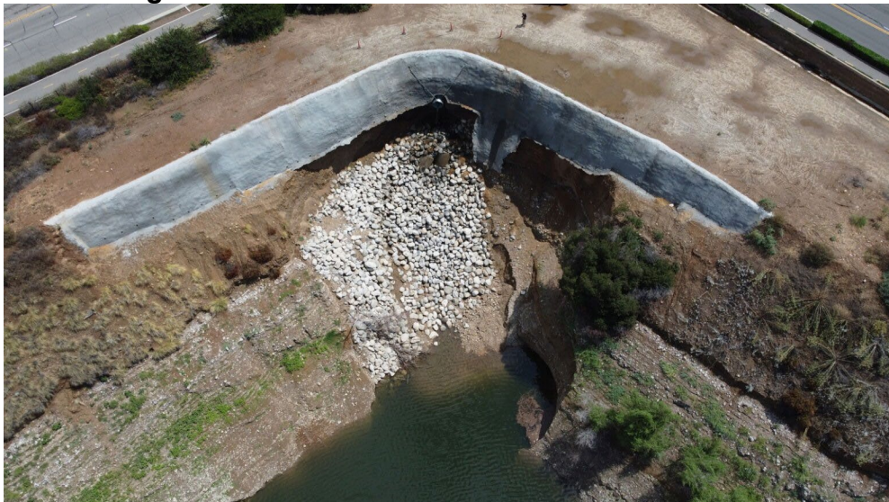
Figure 2 – Soil Nail Wall at corner of Bond Basin
