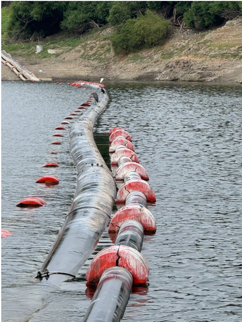
Figure 2 – Pump Station Discharge Pipe and Conduits with Floats
