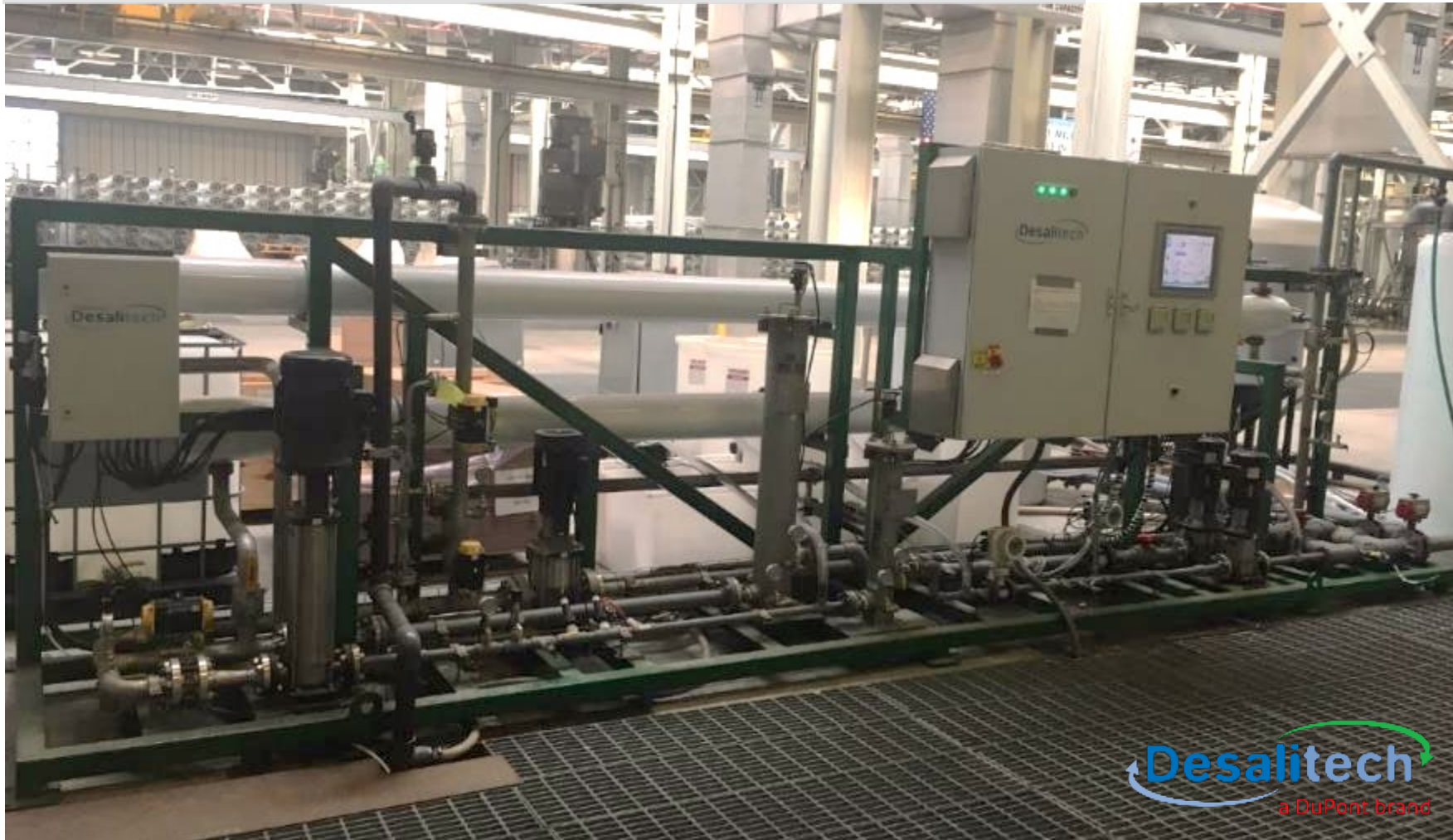
Dupont ReFlex Max CCRO Pilot at AWPf RO Building (2017-2019)
