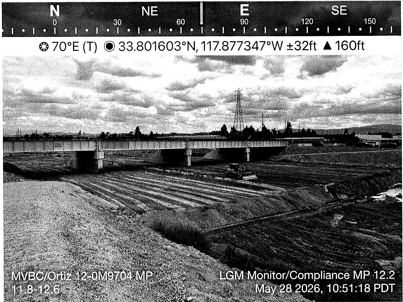
Photo 3: Santa Ana River Reach 4 between the Amtrak rail bridge to the north and Interstate 57 to the south. Photo taken on May 28, 2026, by Lt. Nicholas Molsberry.
