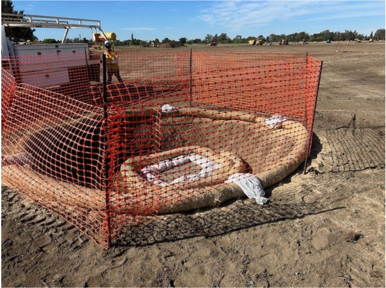
Figure 2: Top of Westbay monitoring well FVM-1 vault after grade change.
