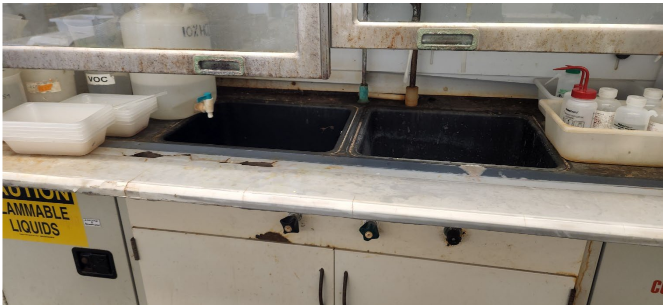
Photo 2: Rusting and corrosion of fume hood internal and external fixtures
