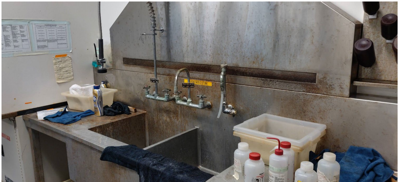
Photo 1: Rusting of fixtures and corrosion damage to faucets at second of three washing sinks
