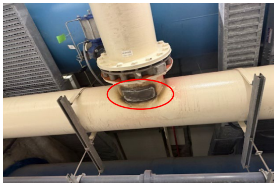
Figure 1 – Welded steel plate repair of pinhole leaks
