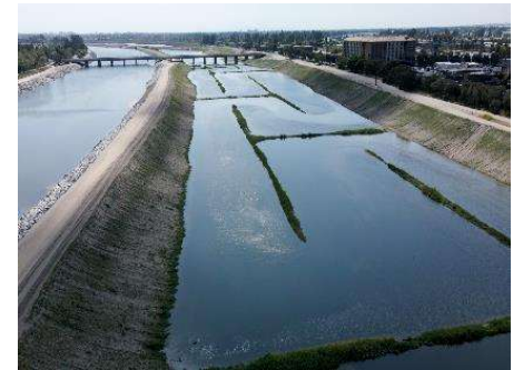
T and L Levees
