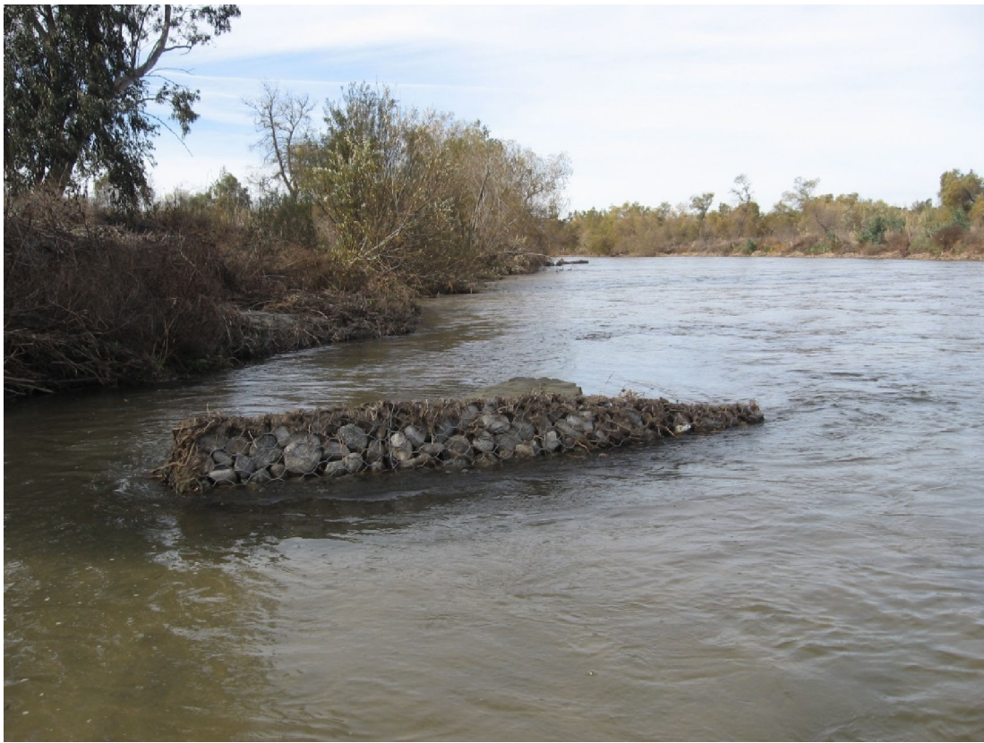
Rock gabion 9 months after installation
