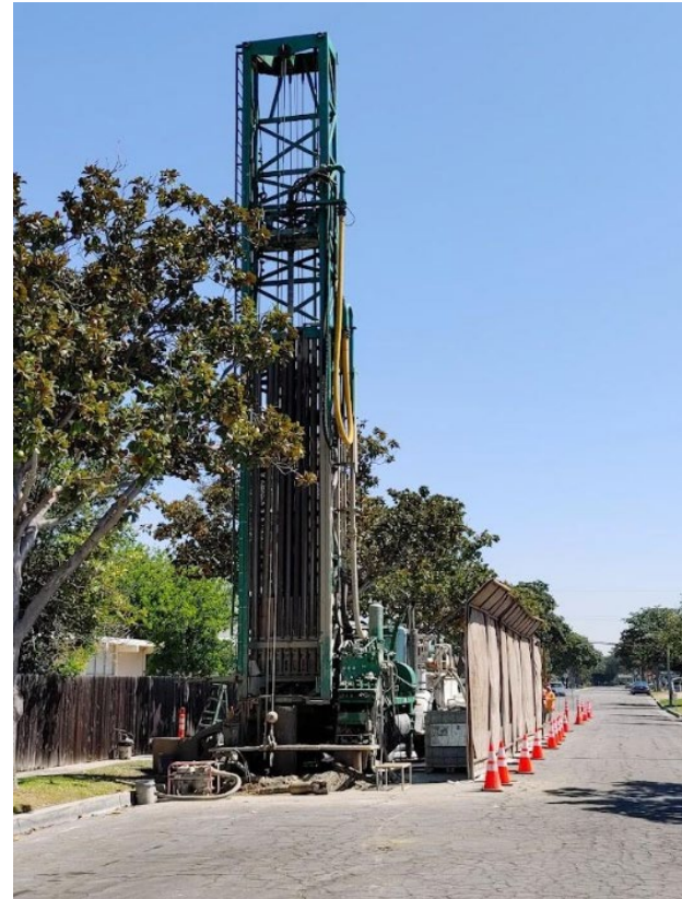
Typical drill rig used to develop a monitoring well.
