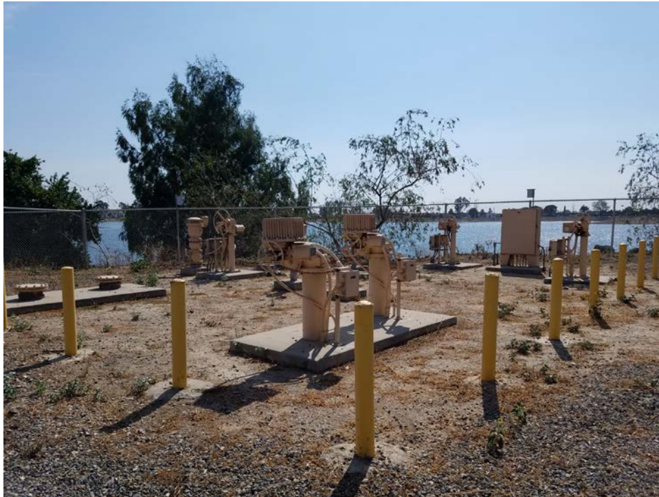
Figure 1: Existing Anaheim Lake Buried Valve Location
