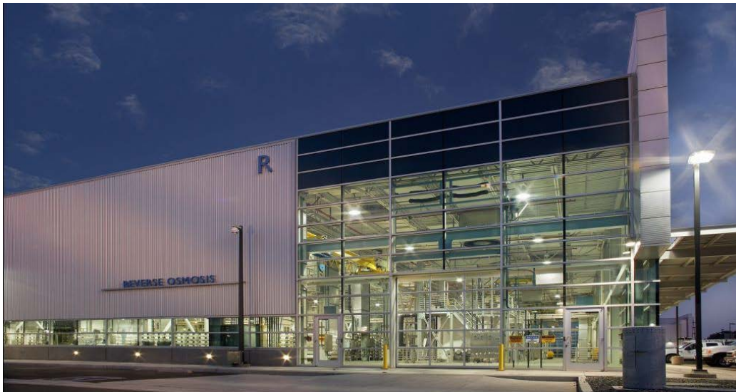
Figure 1-5: GWRS Reverse Osmosis Building
