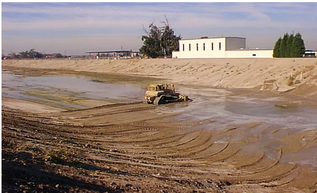
Figure 5-13: Bulldozer in Off-River Channel Removing Clogging Layer
