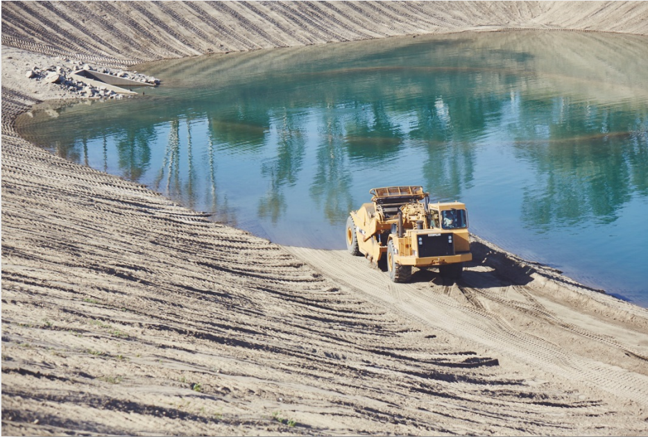
Routine basin maintenance at Anaheim Lake
