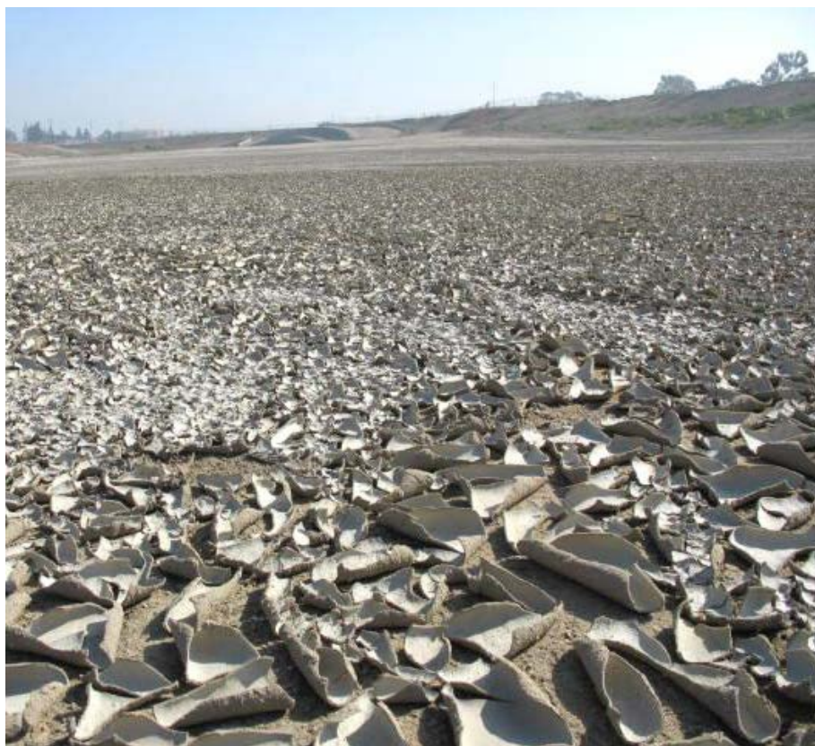
Figure 5-12: Recharge Basin showing Accumulated Clogging Layer
