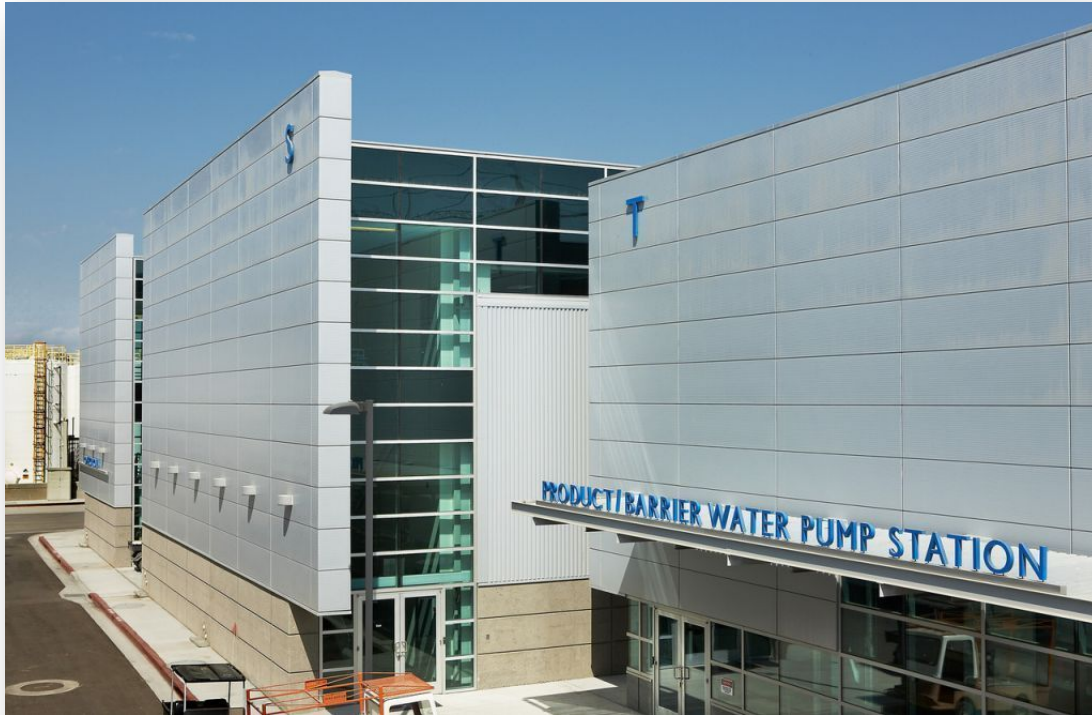
GWRS Water Pump Station and RO Electrical Building
