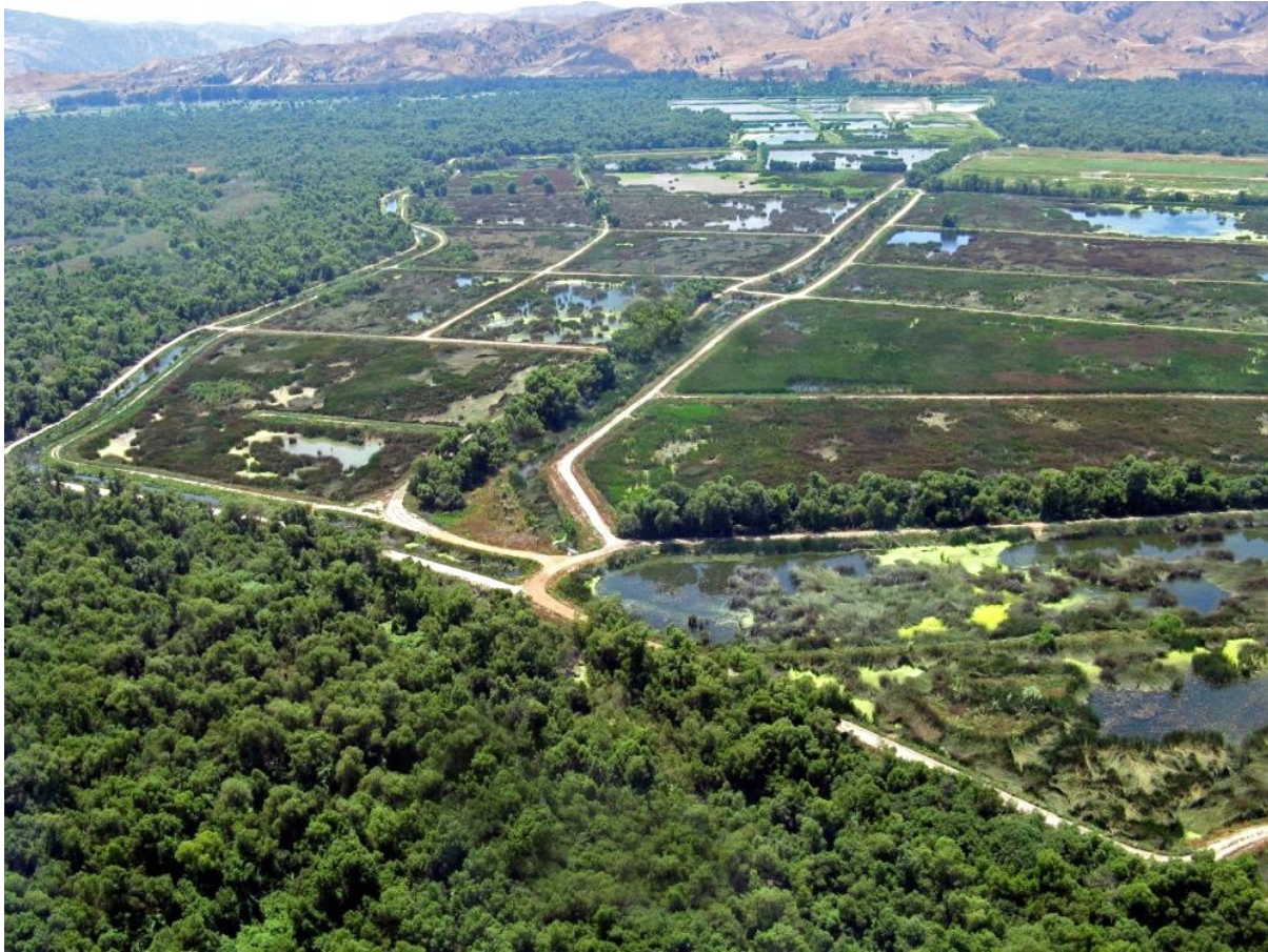
Figure 8-7: Aerial View of Prado Wetlands
