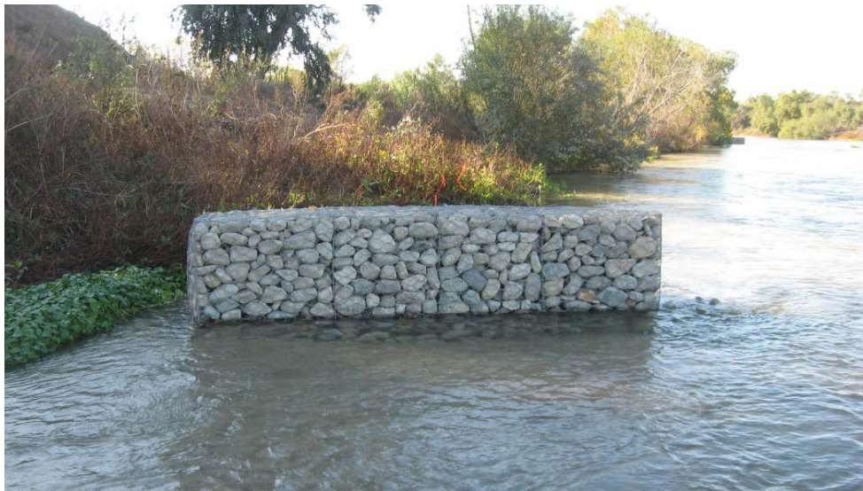
Figure 9-8: Gabion in Santa Ana River Installed to Create Habitat for Santa Ana Sucker
