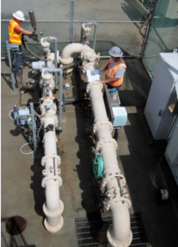
Routine Maintenance of Talbert Injection Wells
