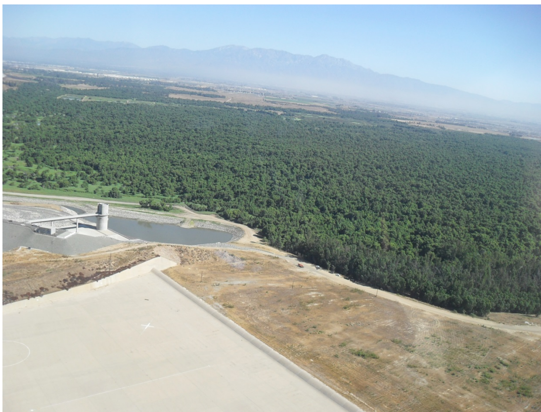
Figure 9-1: View of Prado Basin Looking East with Prado Dam in Foreground
