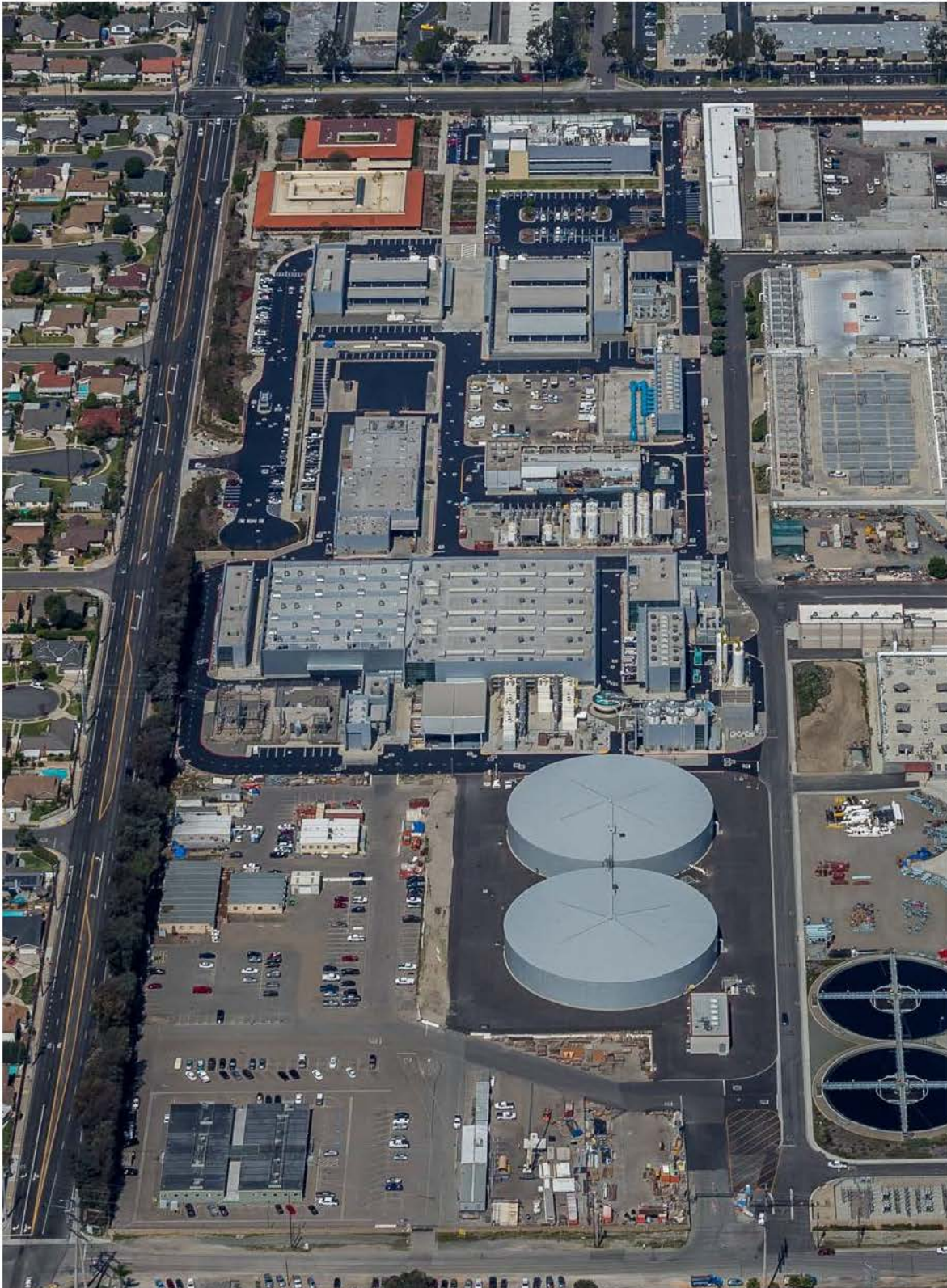
Figure 6-1: Aerial View of the Groundwater Replenishment System
