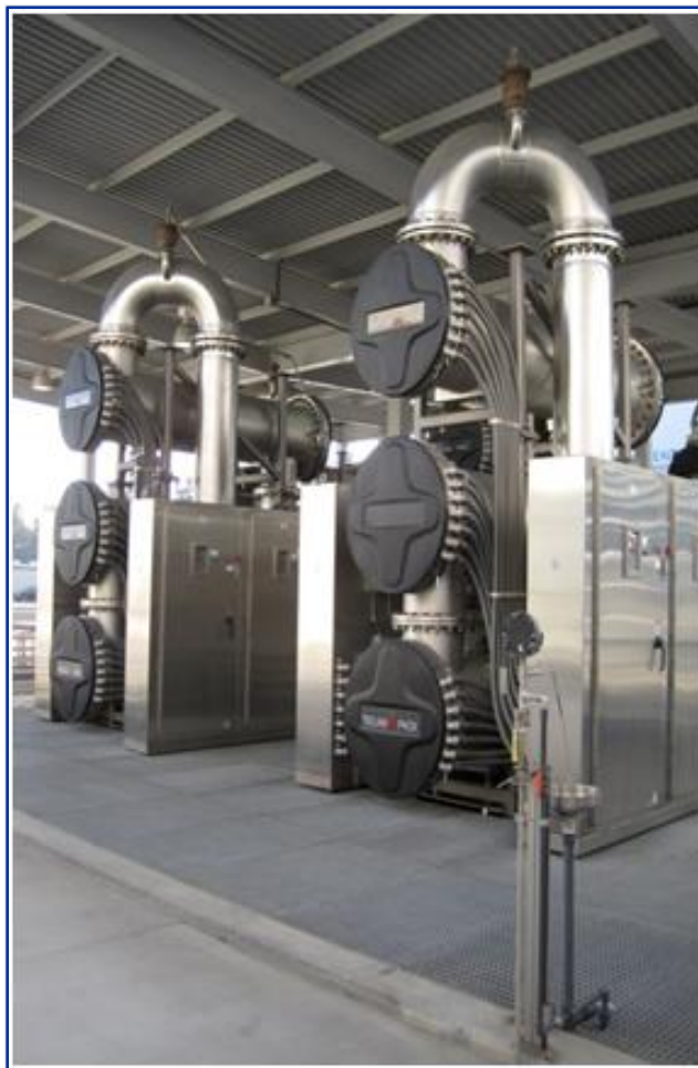
Figure 2-12. UV/AOP System
