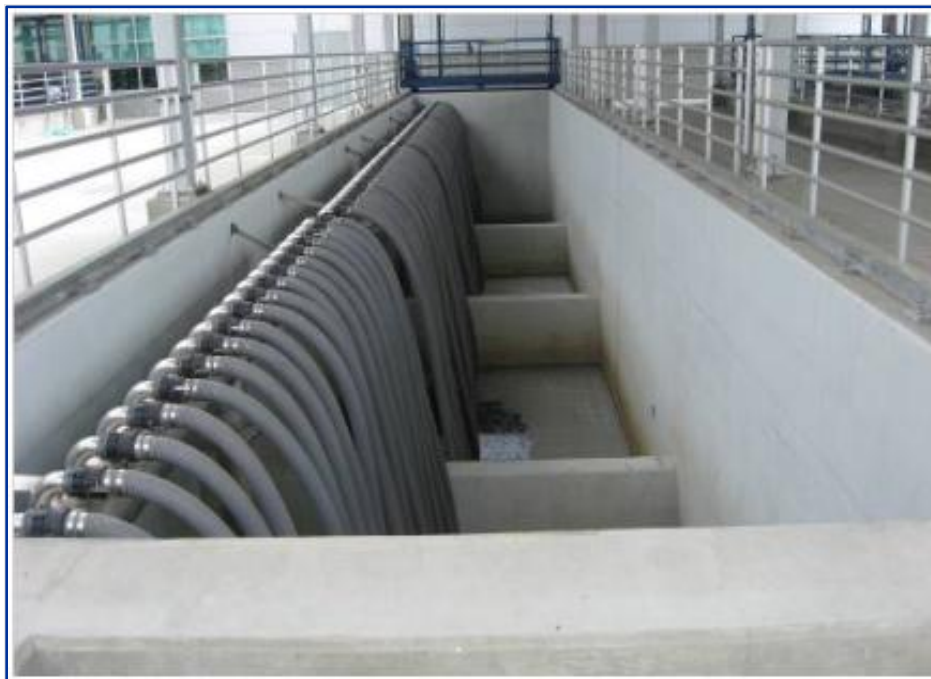
Figure 2-7. MF System
