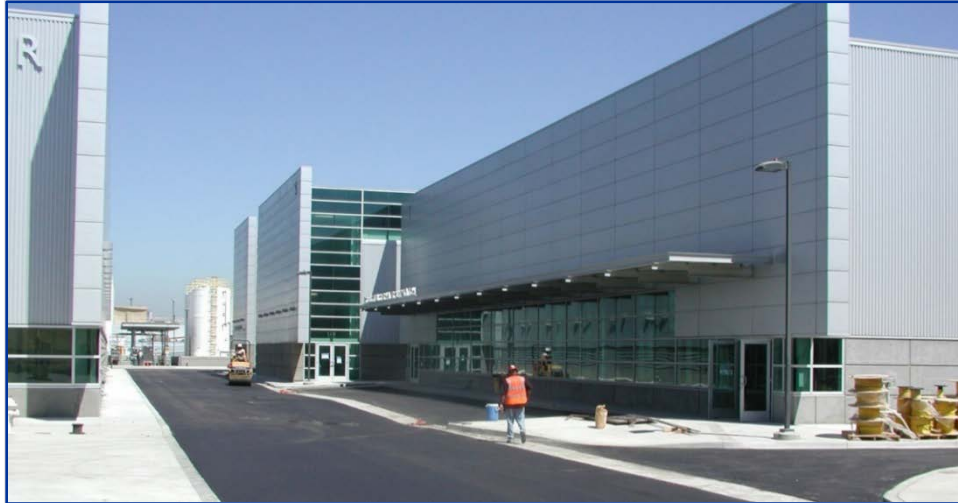
Figure 2-17. Barrier and Product Water Pump Stations
