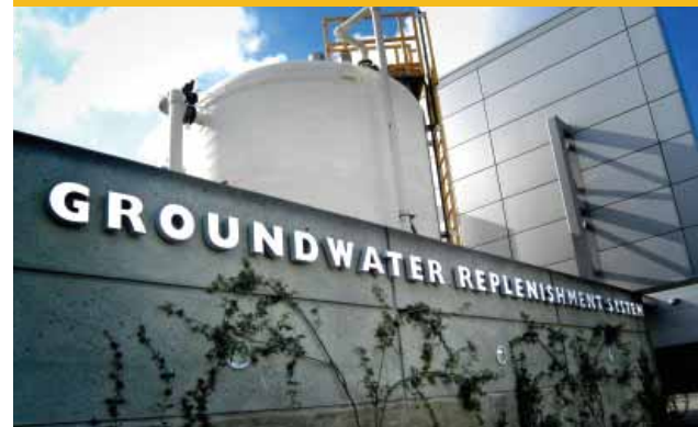
Groundwater Replenishment System (Fountain Valley) Photo: Orange County Water District & Jim Kutzle
