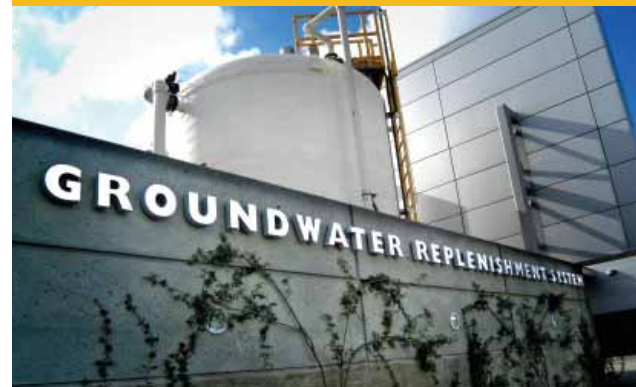
Groundwater Replenishment System (Fountain Valley) Photo: Orange County Water District & Jim Kutzle
