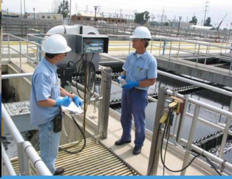
Treatment plant designed for maximum reclamation
