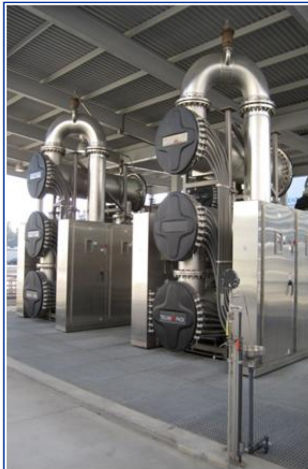
Figure 2-20. UV/AOP System
