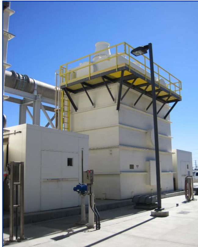
Figure 2-23. Decarbonation System
