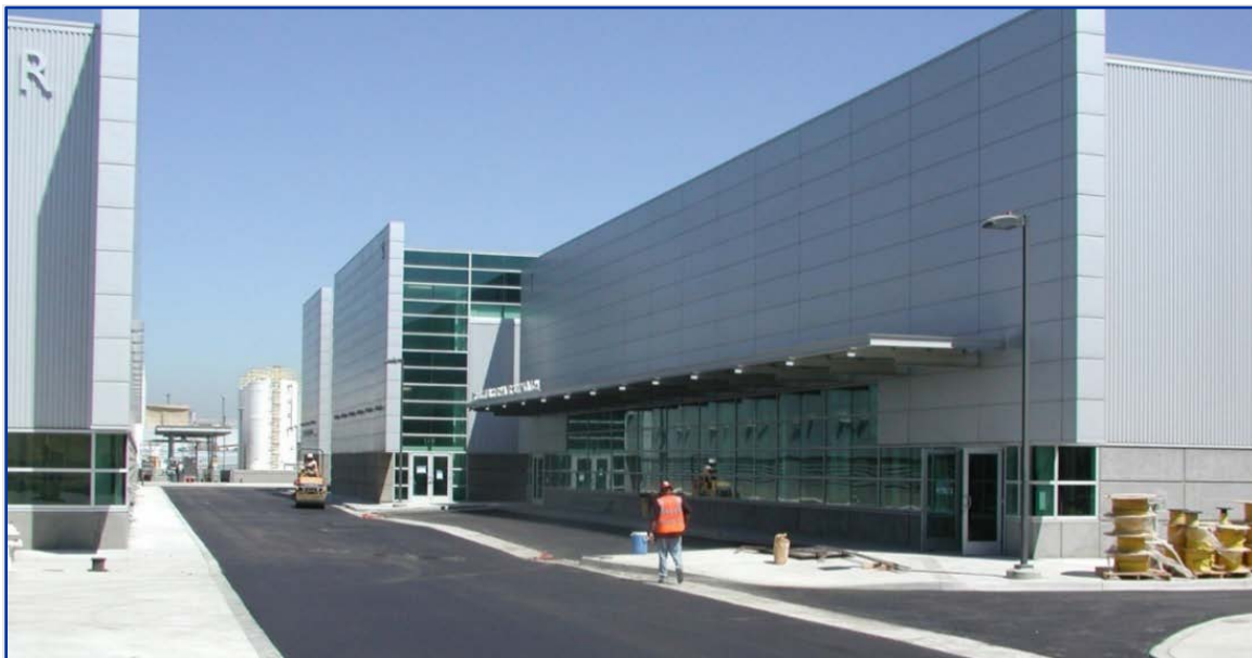
Figure 2-25. Barrier and Product Water Pump Stations
