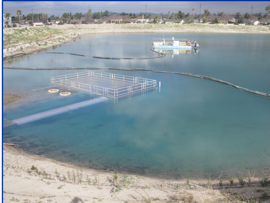
Figure 5-3. Miller Basin with GWRS Purified Recycled Water in 2008
