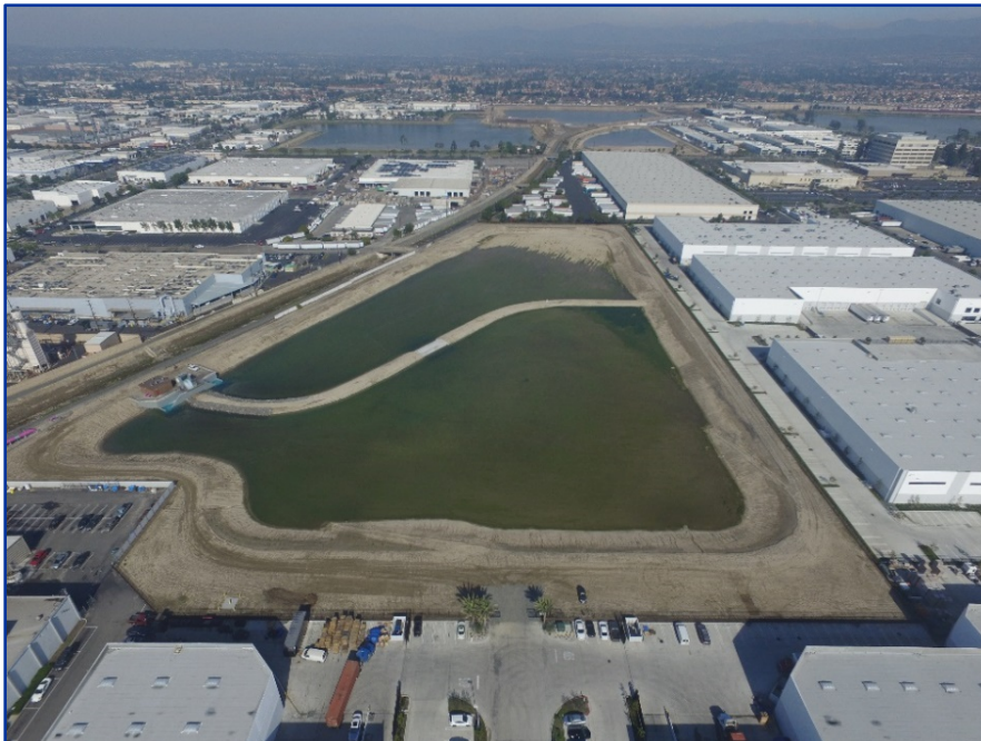
Figure 5-4. La Palma Basin with GWRS Purified Recycled Water in 2016
