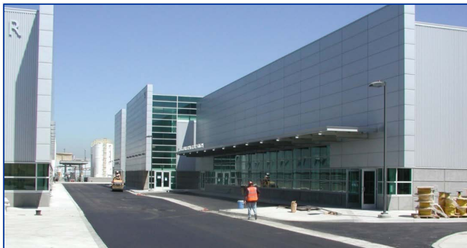
Figure 2-17. Barrier and Product Water Pump Stations
