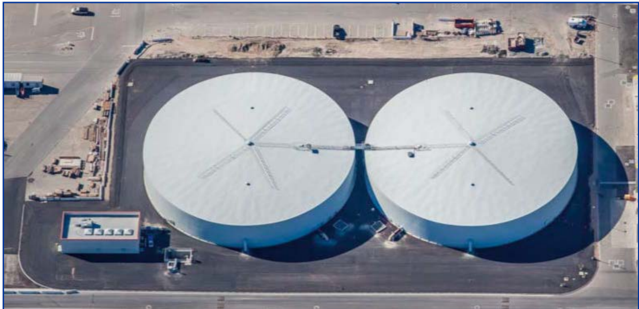
Figure 2-4. Secondary Effluent Flow Equalization (SEFE) Tanks and Pump Station
