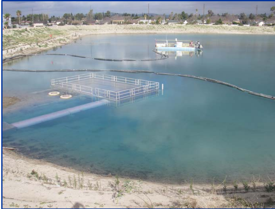
Figure 5-2. Miller Basin with GWRS Purified Recycled Water in 2008
